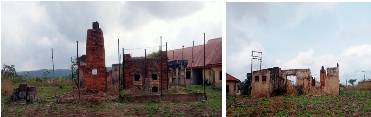
Plate 7: Dilapidated Inyi Pottery Centre/Site built by First Lady, Miriam Babangida in 1990. Source: Fieldwork, 2026
