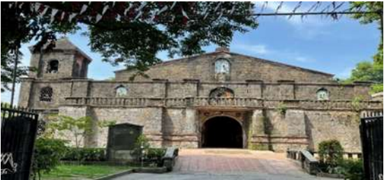
(Front view of the Our Lady of the Pillar Parish-Morong)
