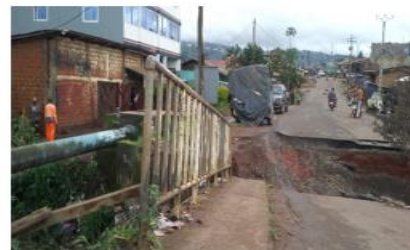
B La Chance bridge
