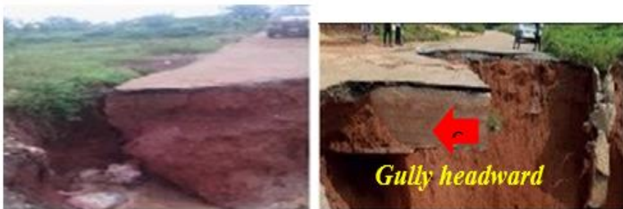
Figure 4: Damaged Roads at Asoro (left) area and UNIBEN (right) by gully erosion
