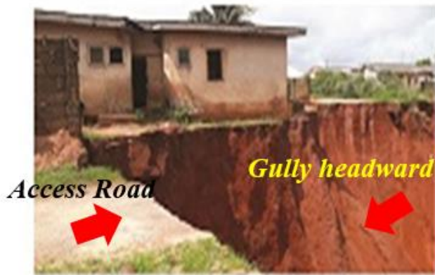
Figure 5: A damaged access road at Iguosa Housing Estate
