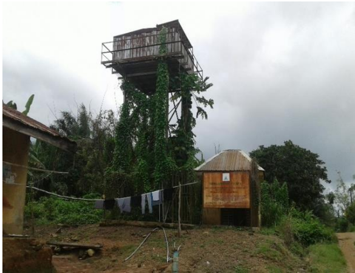
Ile-Oluji FS Federal Govt Water Project
