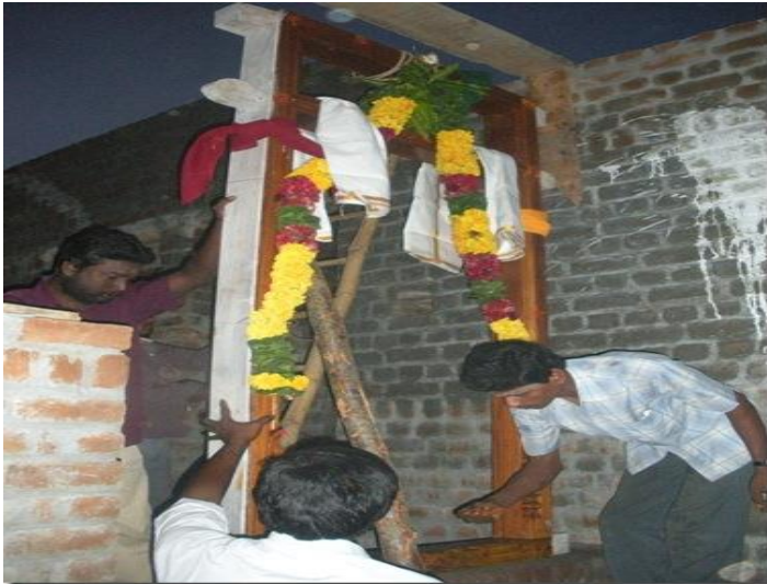
Fig. 8: Erection of the consecrated lintel
