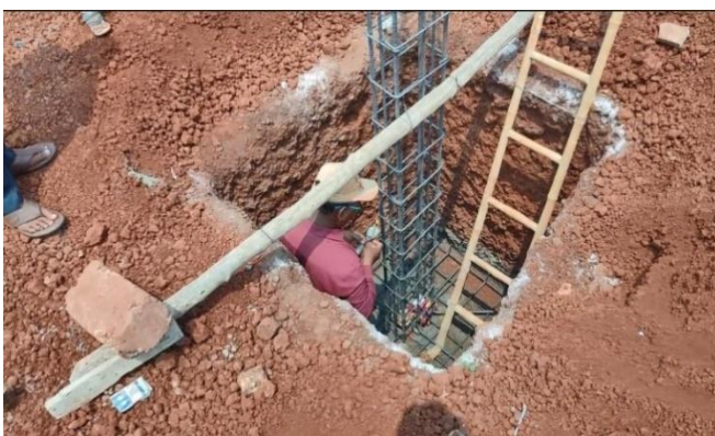
Fig. 4: Bhoomi pooja ceremony of house construction showing foundation deposit of note money, flowers, coconut, burning of incense, relics, ceramic utensils
