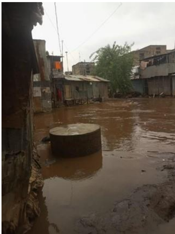
Figure 6: Houses constructed along river bank and on rain drainage area
