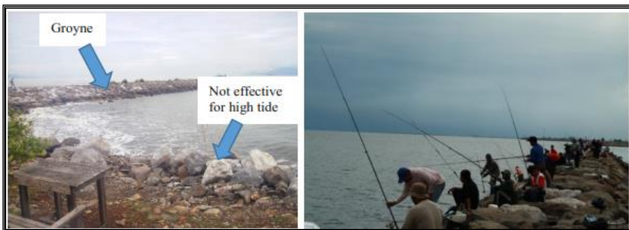
Figure 6. Existing hard protection in the study area.
