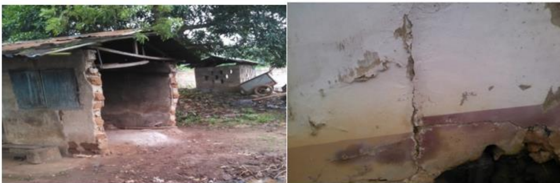
Fig. 5: A=an image of destroyed houses and B=an image showing. These are caused by the blasting of rocks (Ajide & Ajayi, 2015).
