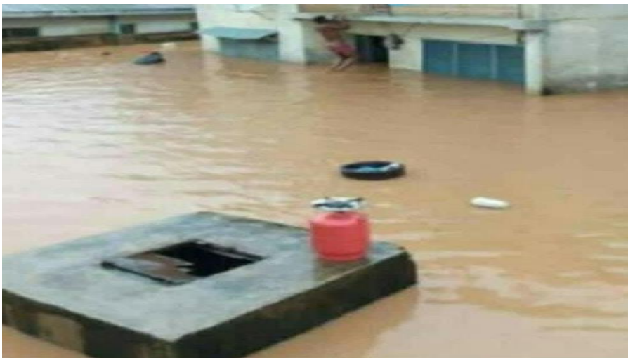
Plate 2: Flood occurrence along Ede Road, Ile-Ife, Nigeria
