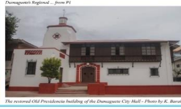
The restored Old Presidential building of the Damaguetas City Hall. - Photo by K. Barabas
