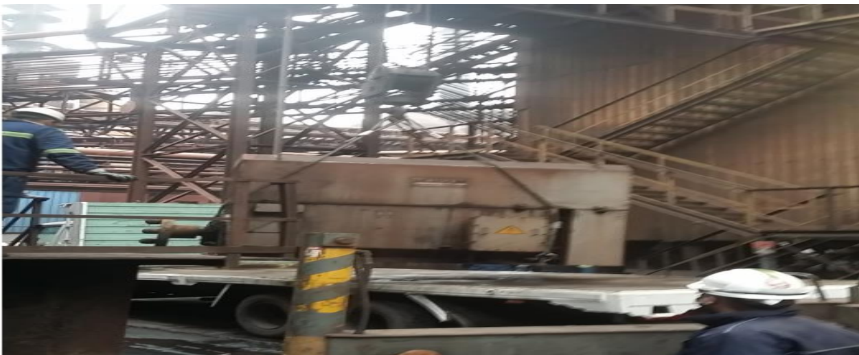
Fig.17 Motor replacement for maintenance
