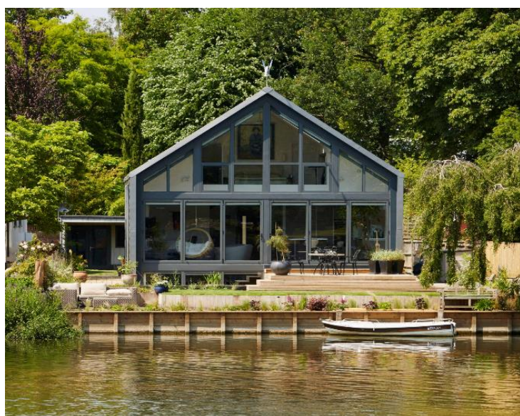
Plate 4. Front view of the Amphibious House, Uk
