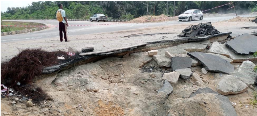
Plate 1: The eroded flexible pavement at the junction to the Cargo Airport along Amassoma Road ( 1 Adedokun, 2022)
