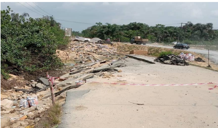
Plate 3: Reconstruction of the failed pavement along Ogobiri - Amassoma Way (Adedokun, 2022)
