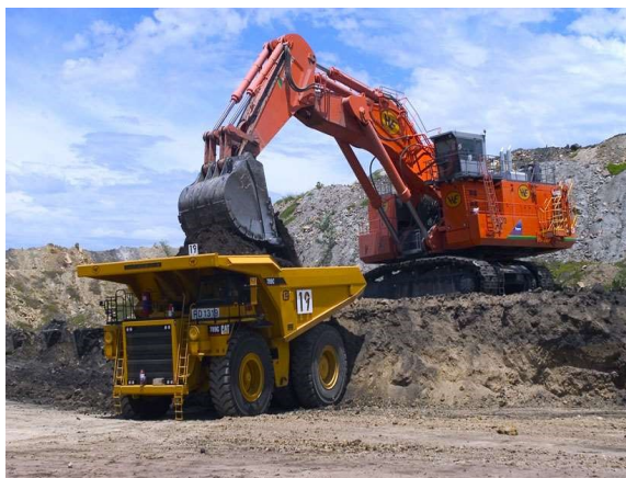
Fig. 2 An excavator in operation - mining
