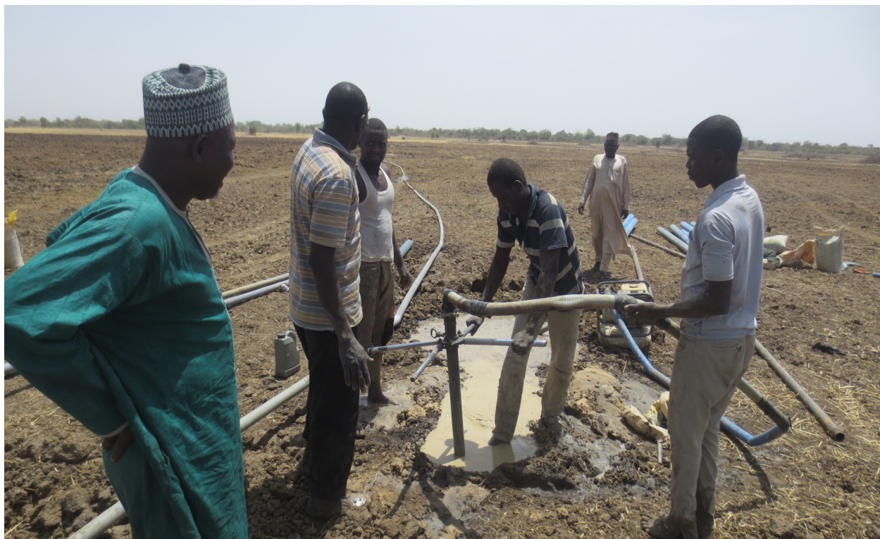
Drilling going on in Dachia, Jakusko LGA, Yobe State
