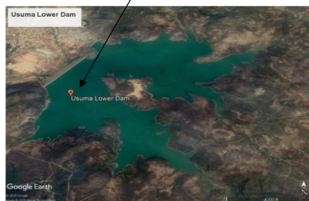
Figure 2 Imagery of Lower Usuma Dam, Abuja
