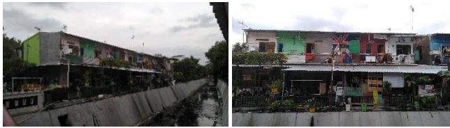
Figure 3. Building a talud along the Pepe River
