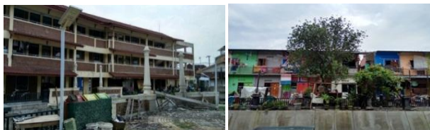
Figure4. PepeRow Houses and Flats in the Pepe River Bank Area
