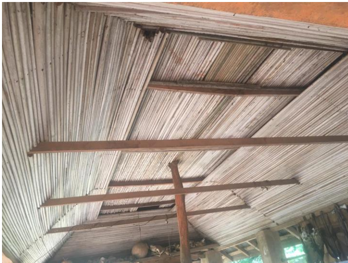
Plate 4.07: Showing a ceiling finished with palm midrib at Nri, Anaocha L.G.A Anambra
