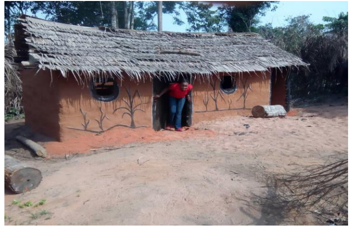
Plate 4.19: Showing a building roofed with thatch roof (palm leaflets) at Ihiagwa ancient Kingdom in Owerri west L.G.A, Imo State
