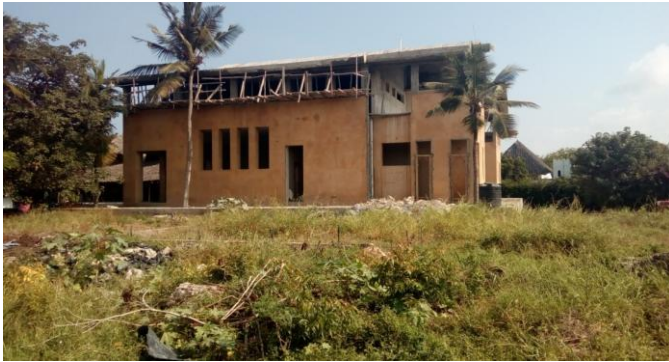
Figure 4. The existing development on Plot 1 at the proposed development project site at Dabaso. Photograph by Mohamed M. Chiguyaso.
