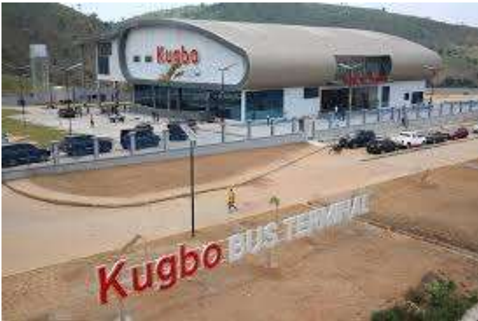
Image 1: Kugbo Bus Terminal as at commissioning in 2025
