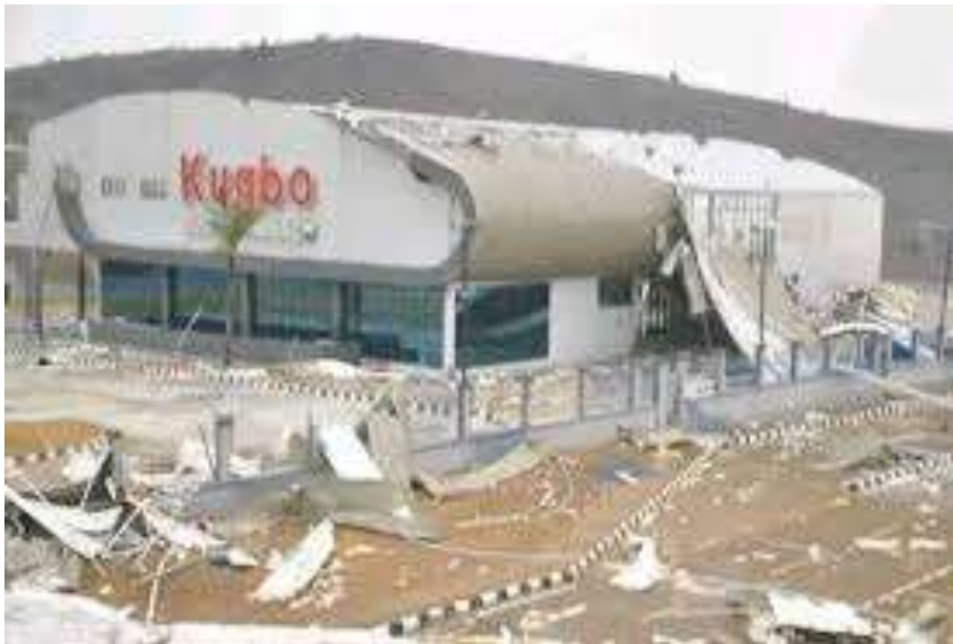
Image 2: Damaged Kugbo Bus Terminal as at 2026
