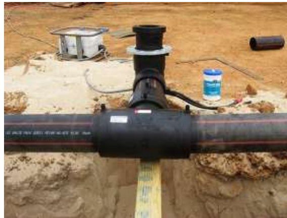
Figure 3. HDPE Pipe Joints
