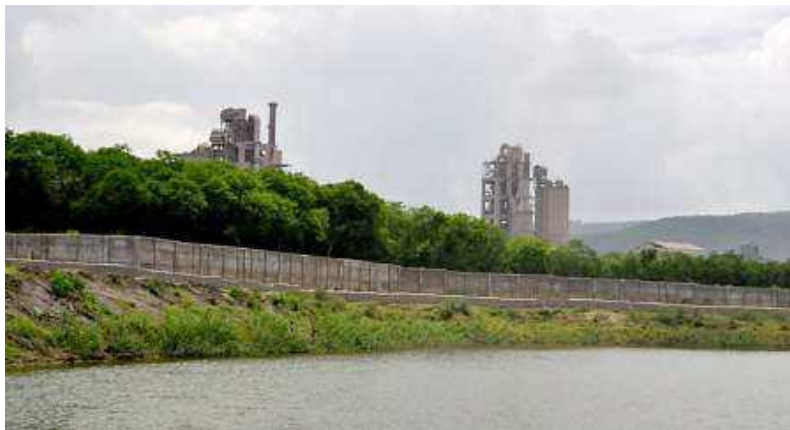
Figure 12: Kymore Cement Works, Kymore, Madhya Pradesh.
