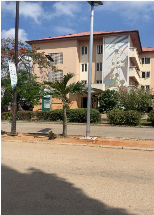
Figure 1: Exterior View of the LASUTH Pediatric Department, Ikeja (Source: Author's Field Survey, 2026)
