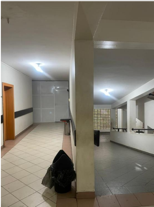
Figure 4: Ramp Providing Vertical Circulation within the LASUTH Pediatric Facility, Illustrating Extended Travel Distance (Source: Author's Field Survey, 2026)
