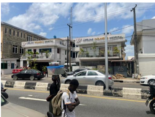
Figure 2: Exterior View of Lifeline Children's Hospital, Surulere (Source: Author's Field Survey, 2026)
